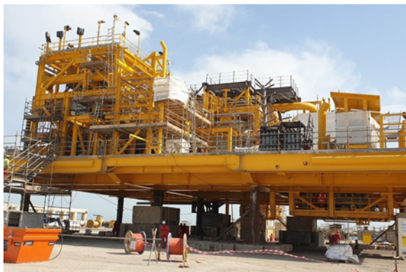
Modules fabrication (April 2022)
