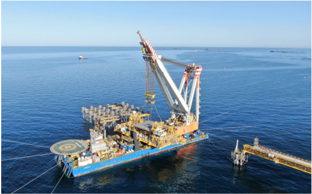
Bridge Jacket Installation
