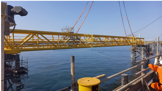
Bridge installation on the mini jackets
