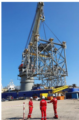
Load-out of the first jacket of Absheron EPS platform
